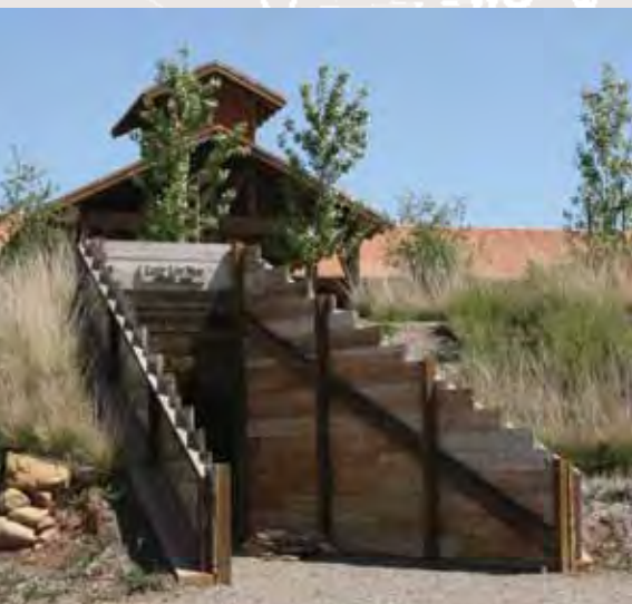
Boy Scout Facility, County of Orange
